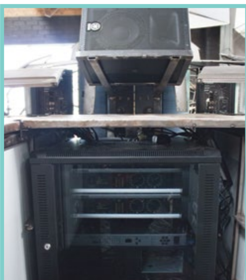
>> Racked up - PC, amps and monitoring
