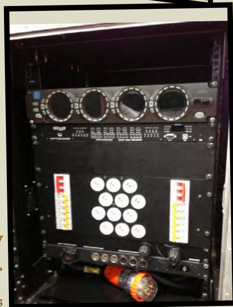
The drive rack for the D&B J System incorporating a Dolby DLP for EQ & Alignment, an Optocore unit which provides a fiber transport solution for control network and AES audio, and a custom 12ch 20A distro for powering the amplifiers. It also shows the 8 way LK multipin which links to the amplifier racks and the fiber bulkhead connectors which link the drive racks together and to the Front of House console.
