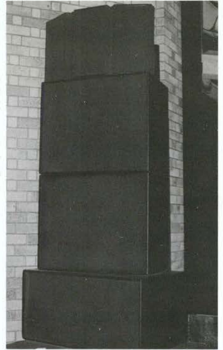
JBL in the theatre: 2 x AP 35 and single 18" sub, (music system) and 3 JBL 4726 Soundpower cabinets (Vocal system)
