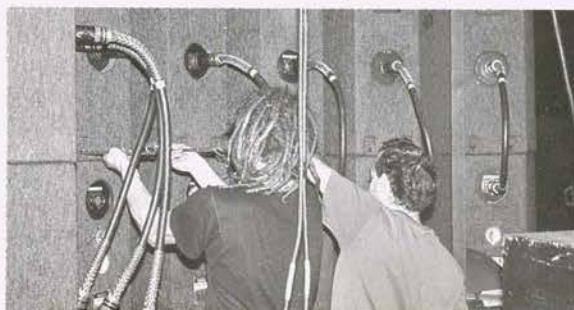
The Prism cabinets form a flush array, joined with steel pins. Cabinets wire together, a column of four is powered by one amp rack.
