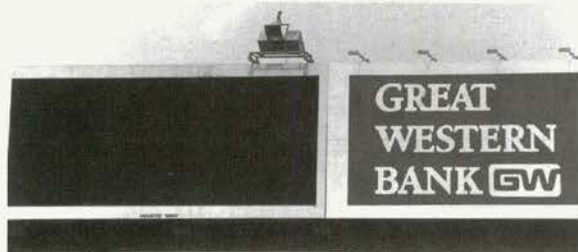
Custom EAW/JBL enclosure at Anaheim Stadium
