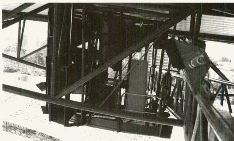
2.5 tonnes of steel platform with a tonne or so of E.V. horns and Neilson's electronics.
