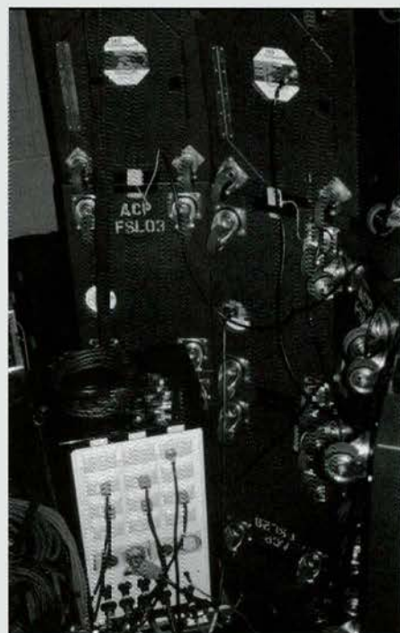
Floodlight, Flashlight, LOW's and the remote power distribution rack. These cabinets were floor stacked to cater to front and rearfill. A cut-back H/Mid cab, underhung from the flown rig can do this. ACP have ordered some.
