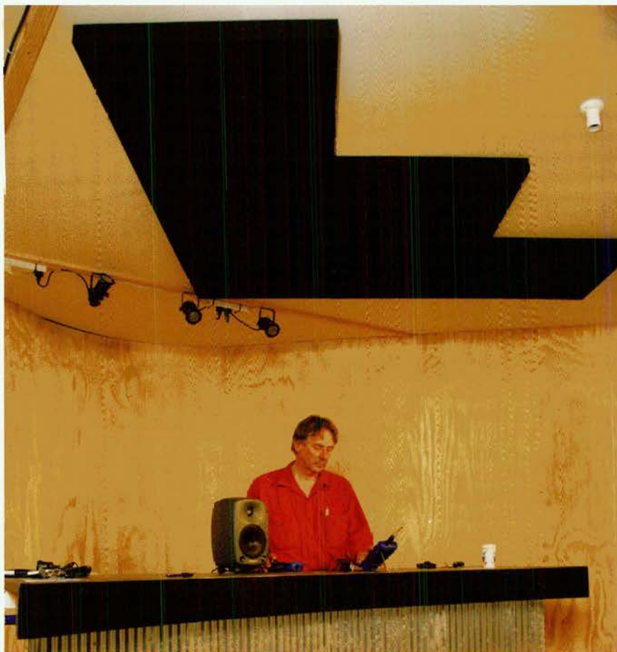
Chris Royal installing primacoustic.
