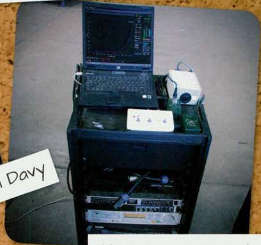
Norwest test rack
