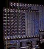
2 x stage DiGiRacks (112 inputs 16 outputs)
