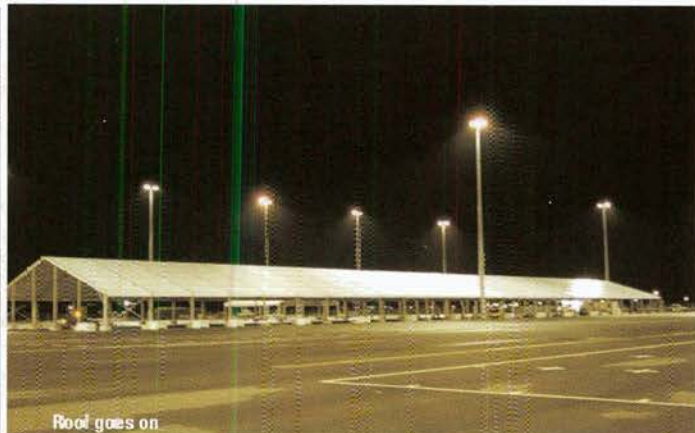
Roof goes on
