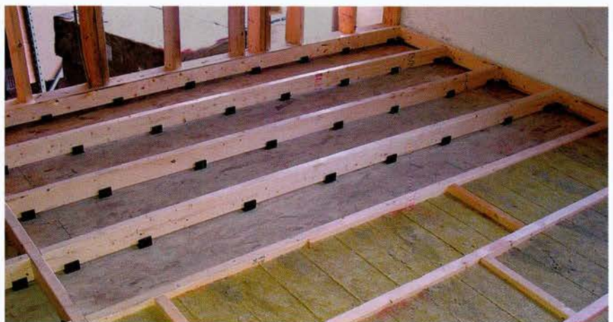
Fig. 2: The construction process. Note how the isolators separate the floor support boards from the "real" floor.
