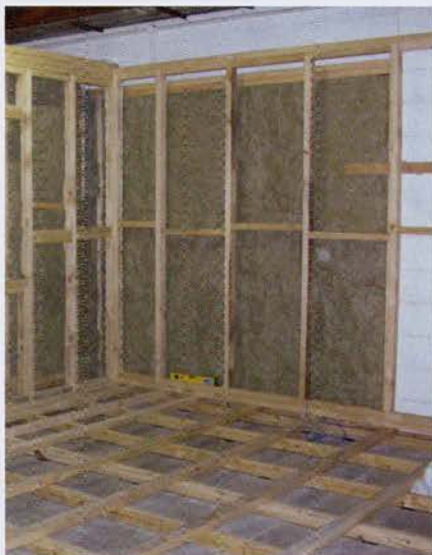
Double everything. Two walls, two floors, and two layers of plaster board on the internal walls.
