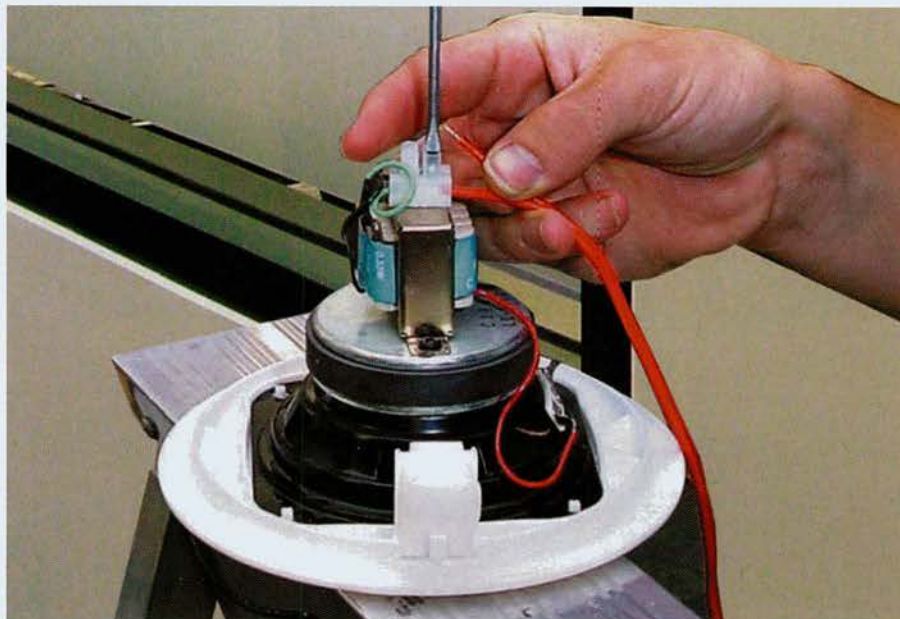
Wiring the primary connection of a 100 volt line speaker's transformer.
