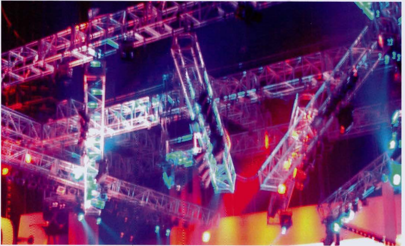
The main 'rock' stage featured a tangled design of chrome box truss suspended from a large mother grid of pre-rig box truss.
