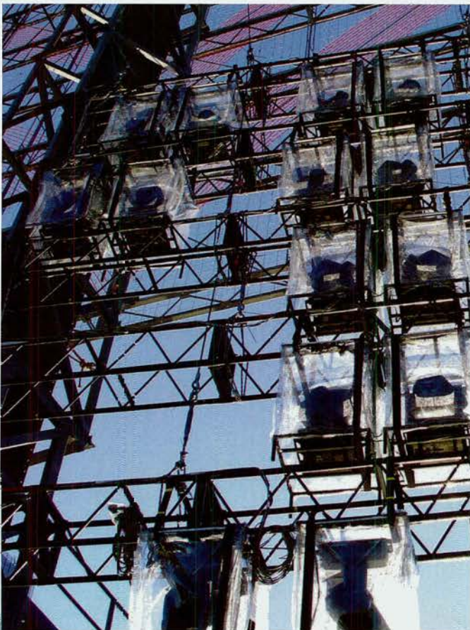
Each light was rigged on a truss and surrounded by a plastic weather shield for operation in any condition.
