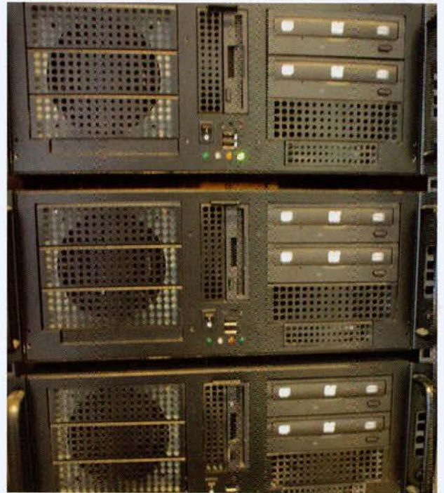
Plenty of stray earth current from a rack like this.
