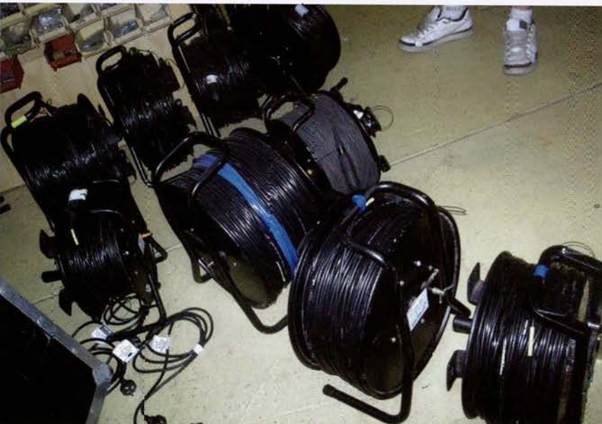
Fibre cables with 5 grands worth of connectors on each!
