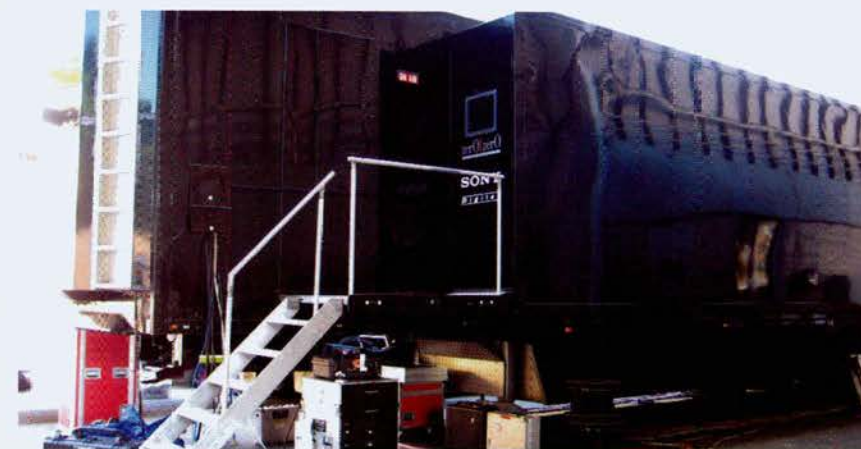
D1 with side expanded - radio base stations under the stairs
