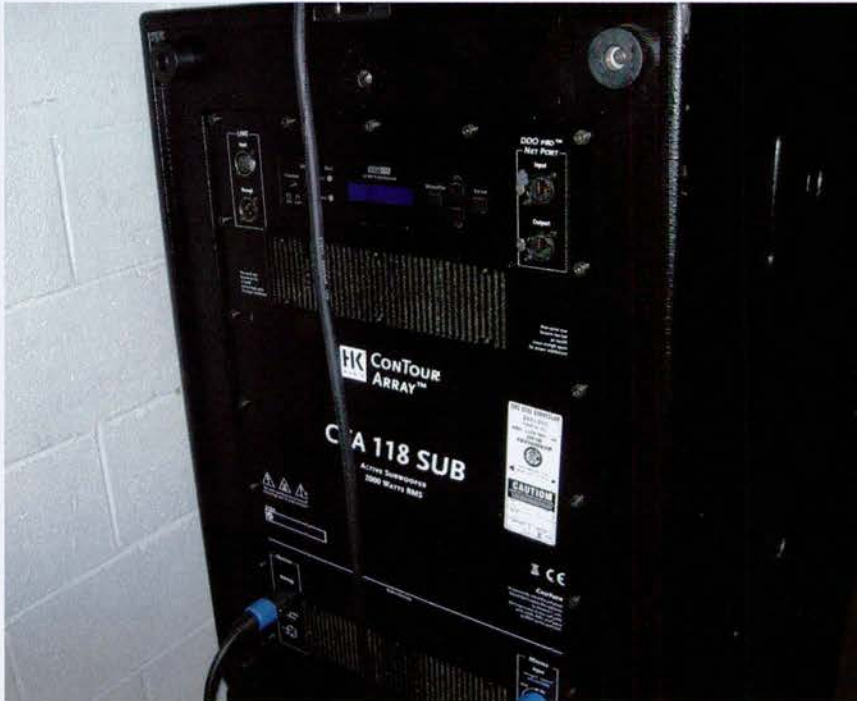
All the processing and amplification for the system gets done in the sub.
