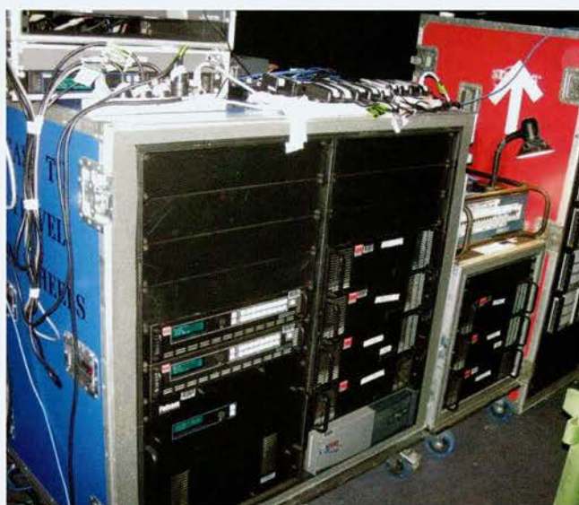
Just a few racks!
