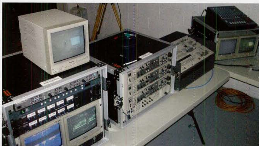
Les bez equipment! This flyaway kit includes a Sony SEG 2550P Special effects generator, Sony Camera Control Units, IRT routers and switcher, and monitoring.
