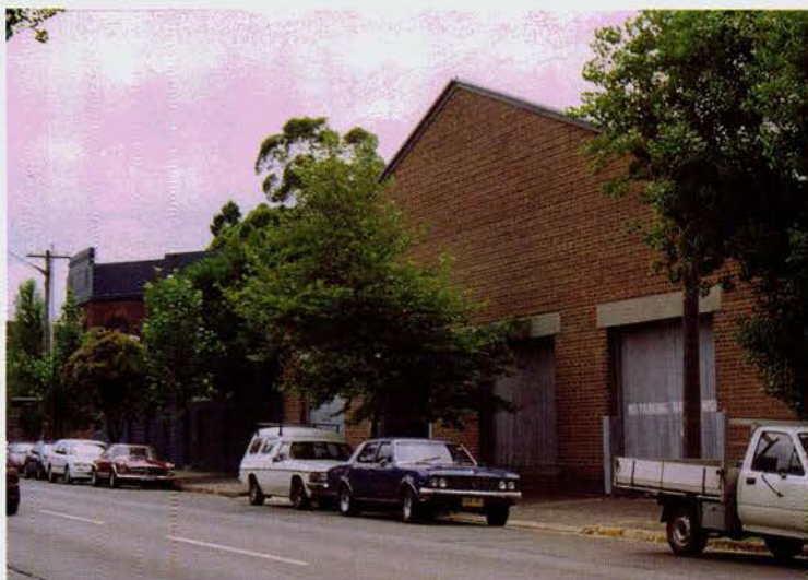
The warehouse (above) is to house an 8000m 2 recording facility
