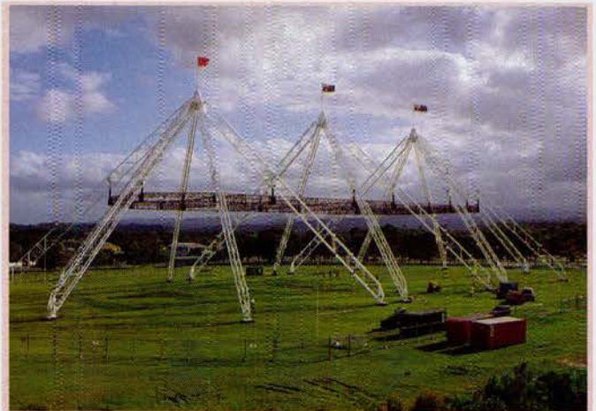
An instant stadium built by Global Events Systems is assembled on the Gold Coast before a sale to Turkey. It's 130 metres long, 64 metres wide and some 40 metres high! 20 GTS chain hoists were supplied by T.C. Hasemer via SCA Distributors in Qld, 16 EM 500 hoists with 25m of lift are mounted inverted at an angle of 45°, & 3 hoists are mounted in each of the 3 spires to haul up the 10 tonnes of membrane tarpaulins. Huge!
