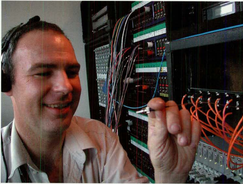
Ian Baldwin with Klotz fibre optic cable
