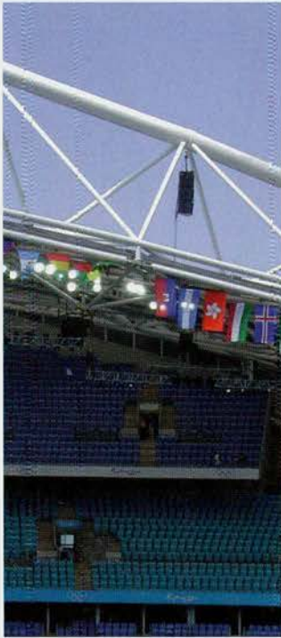
EAW KF750's way above, to cover the North and South (end) stands
