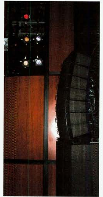
(above) DV-DOSC Line Array as it is set up in the Lyric at Star City. There are left and right stacks of 7, as shown atop 2 bass bins, plus floor left, right and centre arrays.
