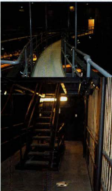
(bottom) Backstage Stairs - The stairs that connect the various gantry levels surrounding the stage have two very logical design features. Firstly, they are stairs and not a glorified ladder - so you can ascend/descend facing the direction you are going and also carry a full load while you are doing it. Secondly, the rungs are wooden - making it possible to use them quietly.
