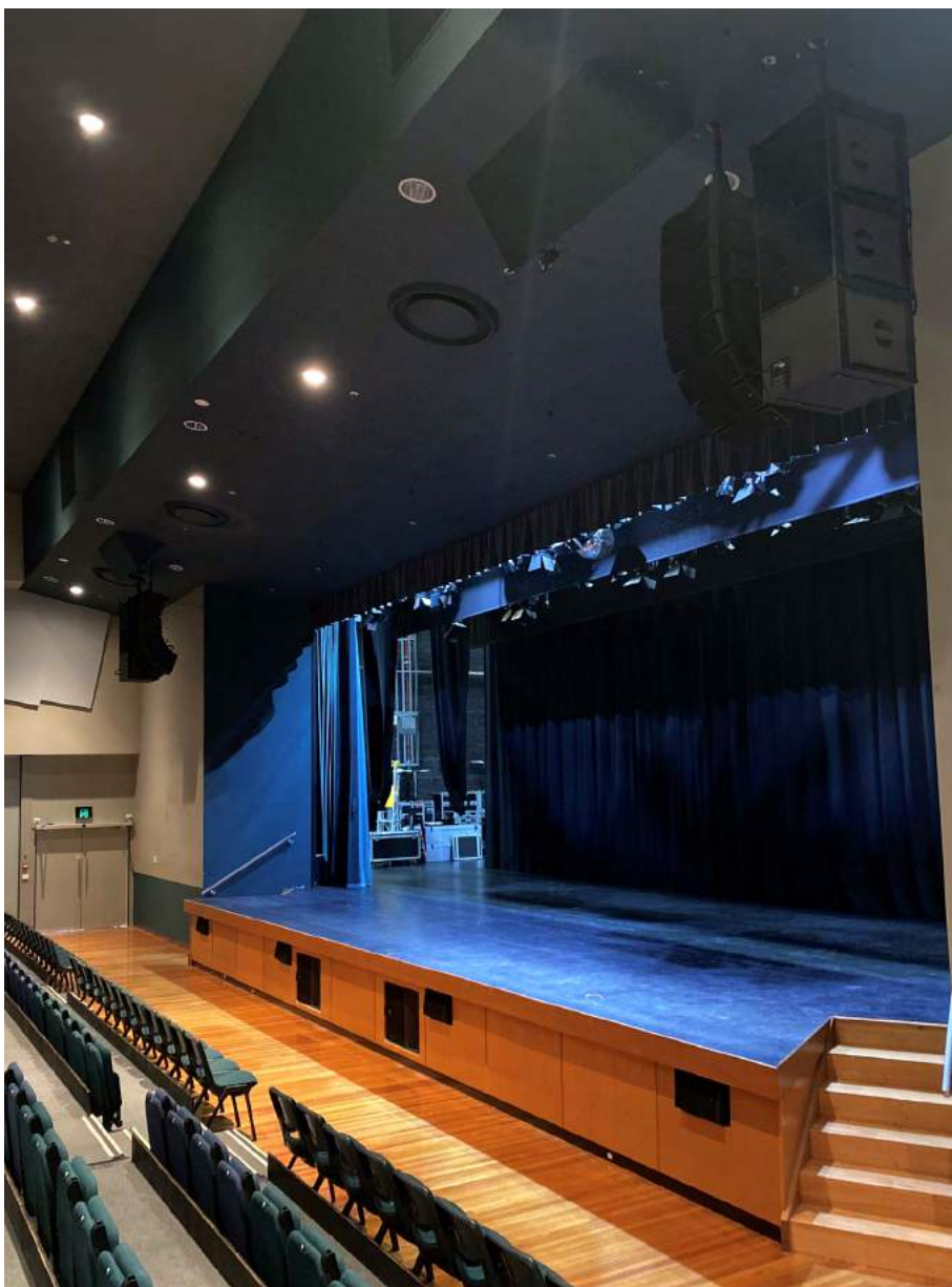
The new PA system consists of eight L-Acoustics Kiva II enclosures per side flown next to three SB15m subwoofers. Underneath the stage are a pair of KS21 subwoofers.
