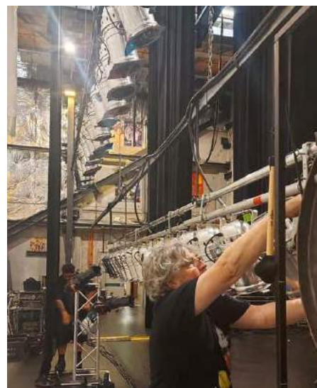
Michael Knapp, Production Manager, The Green Room Ltd. Focusing 18 x 6 bars of Par 64 cans along with the Kiri te Kanawa Theatre house rig (Aotea Centre, Auckland)
