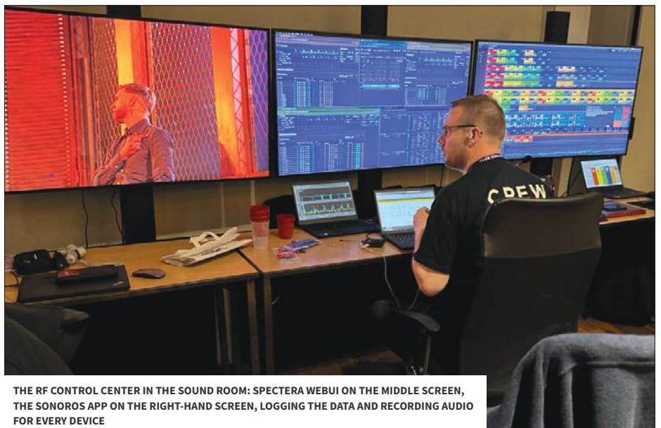
SIX RACK-MOUNTED SPECTERA BASE STATION WERE ON DUTY IN THE SOUND ROOM, FOUR WERE ACTIVE, ONE USED FOR SCANNING, NO. 6 WAS A SPARE
